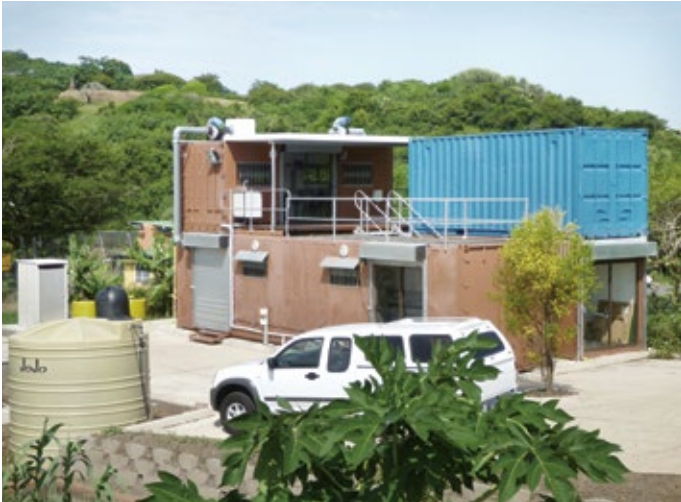
Figure 3: At the Newlands-Mashu Field Test Site, multiple nutrient recovery technologies can be tested under realistic conditions. Besides the urine treatment plants, the containers host an analytical laboratory and a field office.
