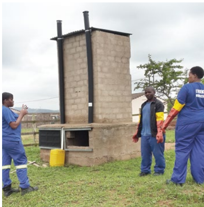
Figure 1: Urine collectors measure and record the collected urine volume before they pick up the yellow jerry can from a urine-diverting toilet in eThekweni.
